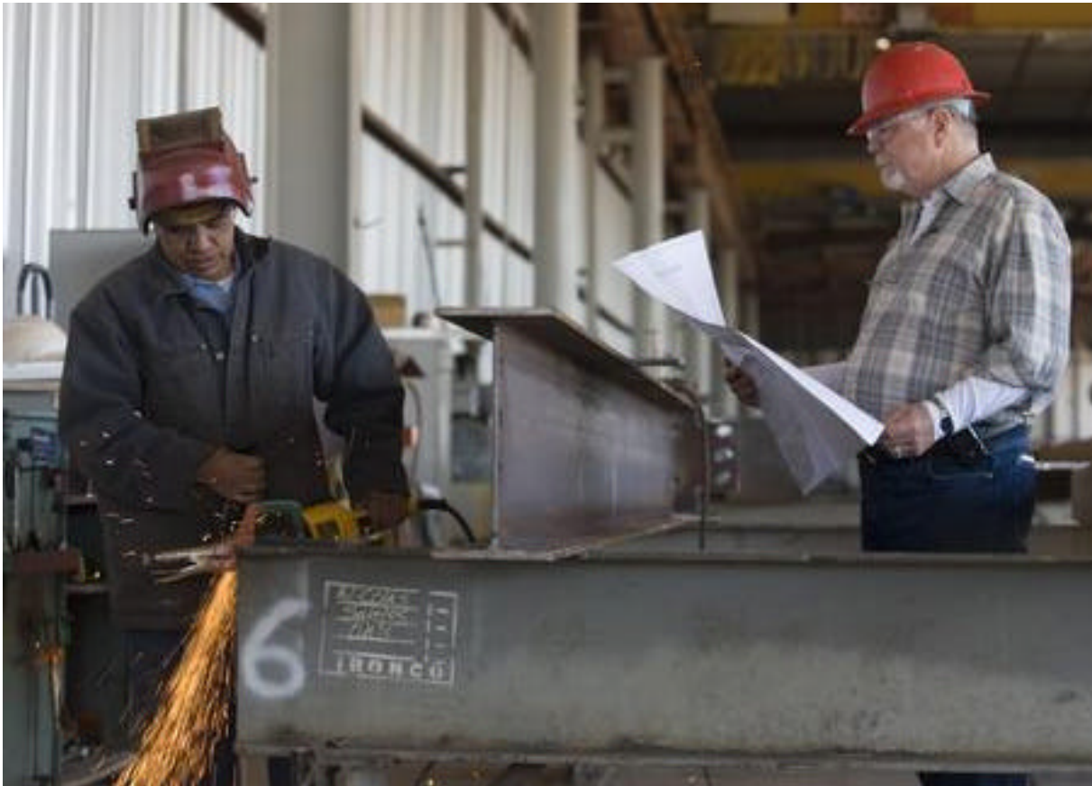
Christine Keith/The Arizona Republic Ironco welder Nicolas Santos (left) fits braces while company owner Sheridan Bailey looks over a layout plan. In December, Bailey formed Arizona Employers for Immigration Reform to voice concerns of business owners.
